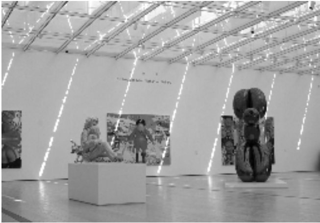
Figure 4 Unfiltered light entering third floor galleries
