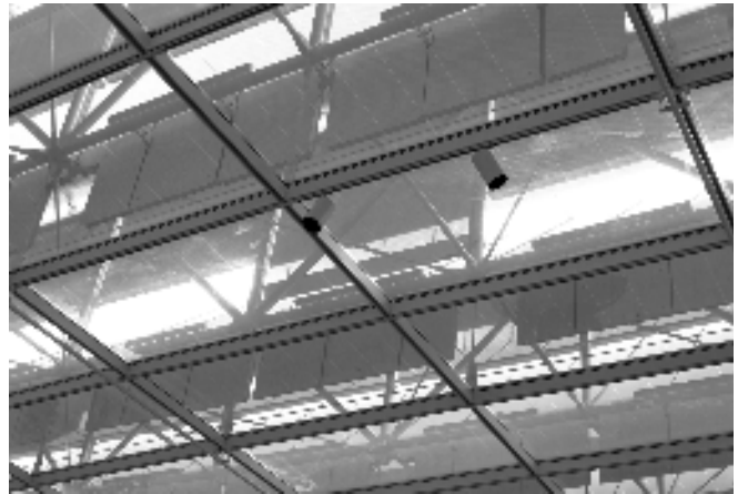
Figure 1 Third floor gallery ceiling construction
