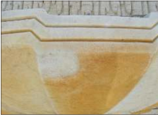
Figure 6. A test cleaning after two minutes of gel application
