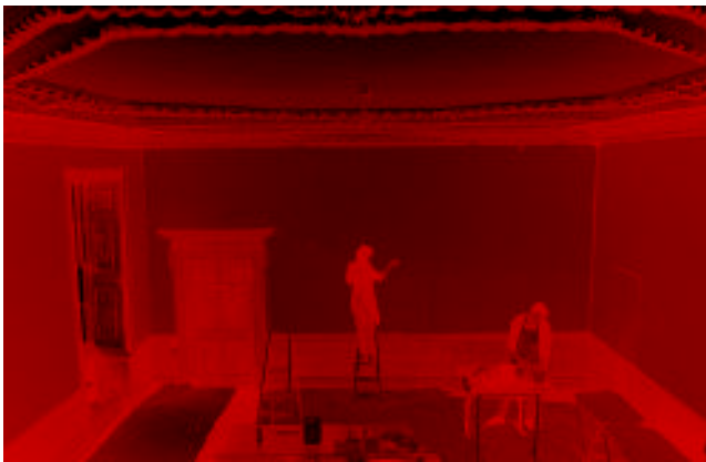
4. The Ukekake ('cushion' or 'pocket') layer being applied to the first layer of Japanese paper in quarter sheets.
