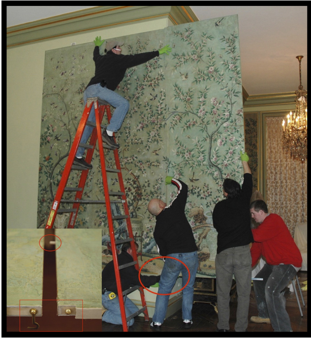
Fig. 10. Newport panels secured within moldings with detail of panel alignment hardware, photo Studio TKM.
