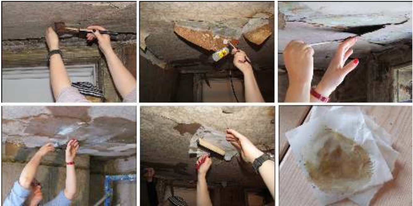
Fig. 8. Process of wallpaper stabilization using Tri-funori includes cleaning, consolidating, re-adhering, saturating, flattening, and cleaning.
