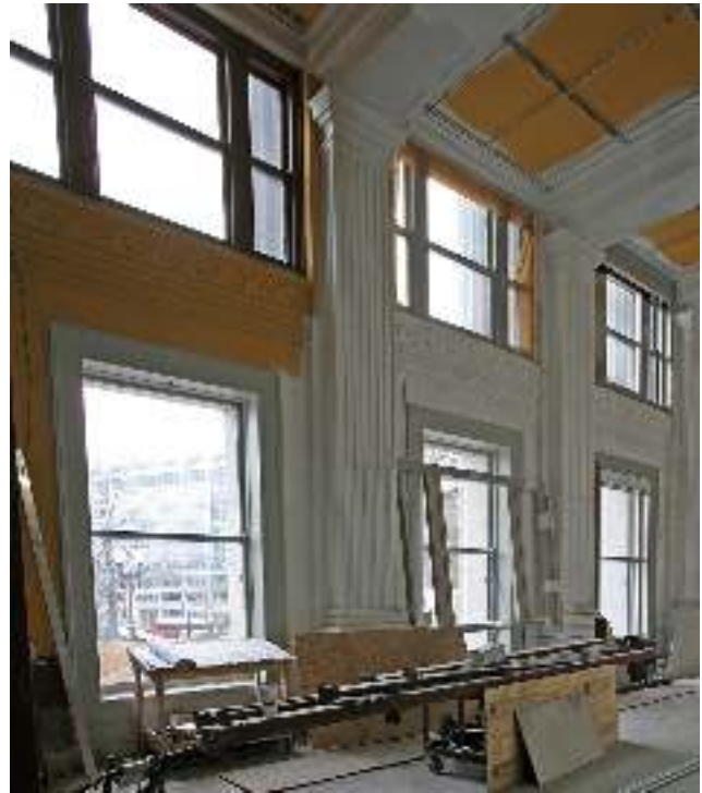
Fig. 8. South facing historic windows.
