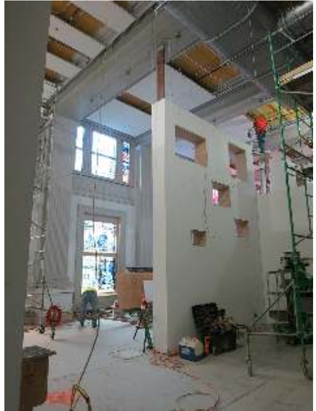
Fig. 7. Constructing barrier walls to block sunlight.
