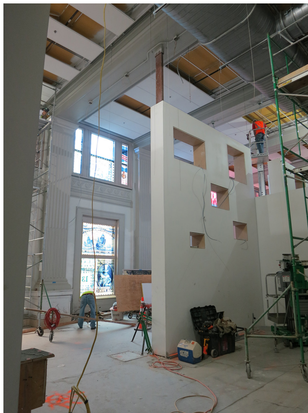
Fig. 7. Constructing barrier walls to block sunlight.
