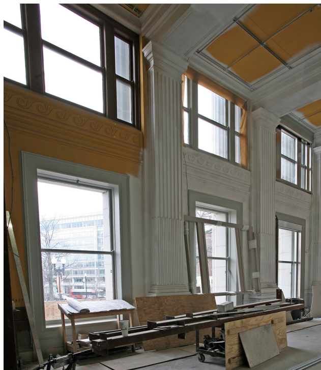
Fig. 8. South facing historic windows.
