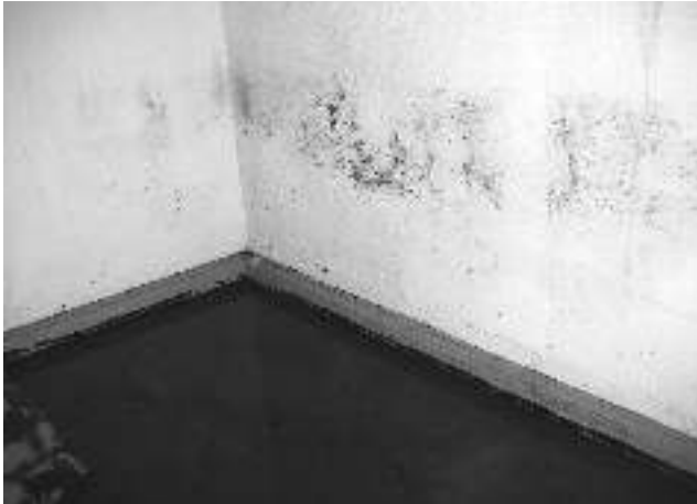
Fig. 1. Staining on stairwell walls indicating the highest level reached by floodwaters.
