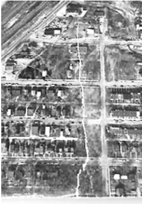
Fig. 3. Improperly aligned mend
