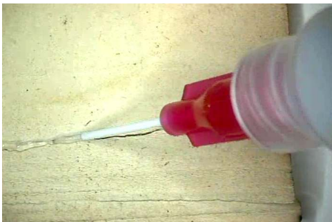
Fig. 6. Application of thicker fluid (wheat starch paste) using flexible tip.
