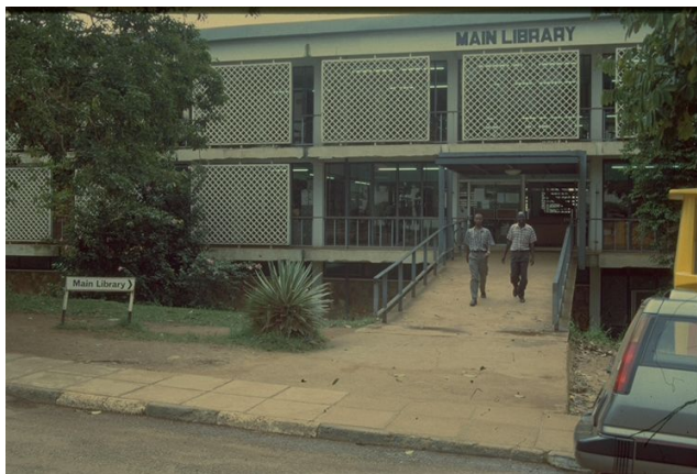
Fig. 1. Makerere University's Main Library building, front view. Notice the dust road that leads to the entrance, allowing a thick red dust to enter the library and settle on the shelves and books, disfiguring the library holdings and potentially causing abrasion. (Photo by E. Kissel, 1999)
