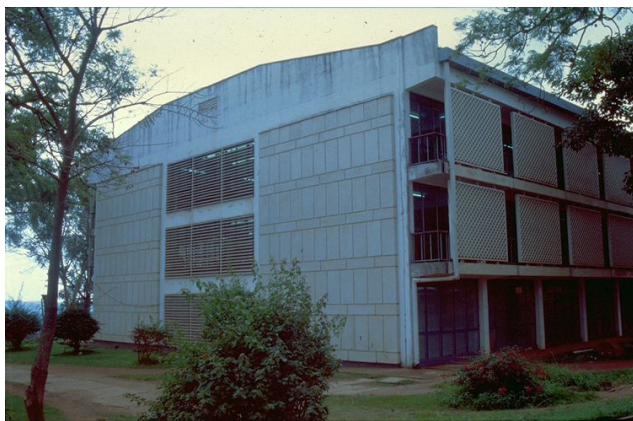
Fig. 2. MUKL main building, side view. The construction allows the air to flow freely through the building, as most of the windows located behind the lace-like concrete panels are opened. (Photo by E. Kissel, 1999)
