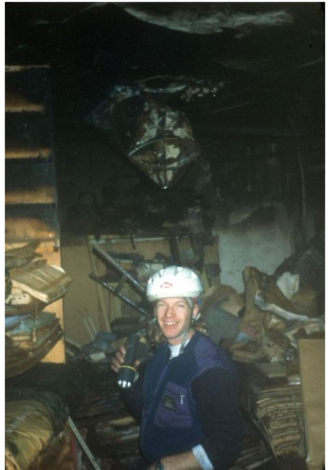
Fig. 3. Water damaged inventory
