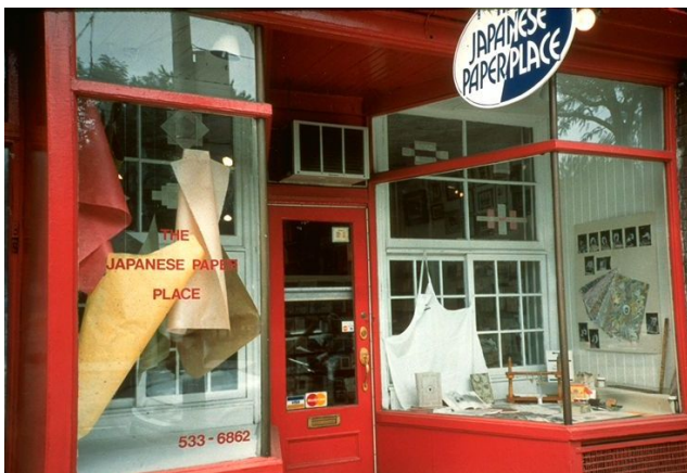
Fig. 1. The store front before the fire
