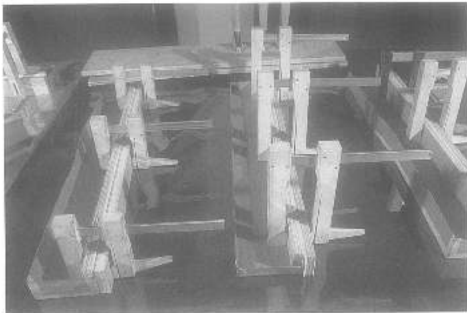
fig. 32. Reshaping and drying cockled sides
