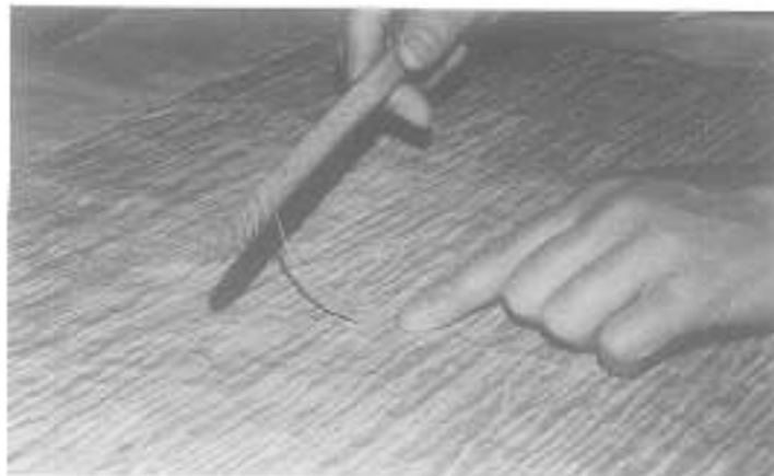
Fig. 12. Apply over creases and tears
