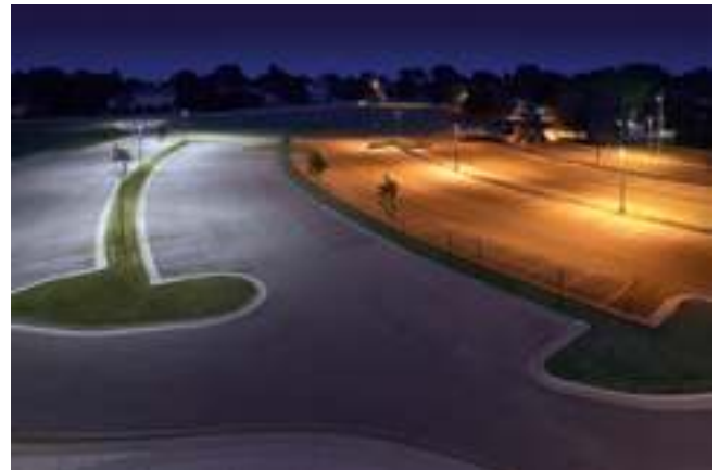
Figure 2. Installation of LED parking lot lights (left) compared to HPS lights (right) shows the difference in color appearance and distribution. Photo credit: Beta Lighting.
